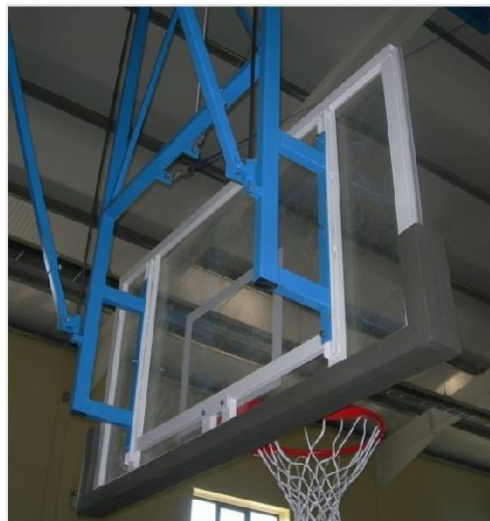
Fig. 2 Drop down goal support structure example
