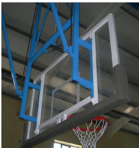
Fig. 2 Drop down goal support structure example
