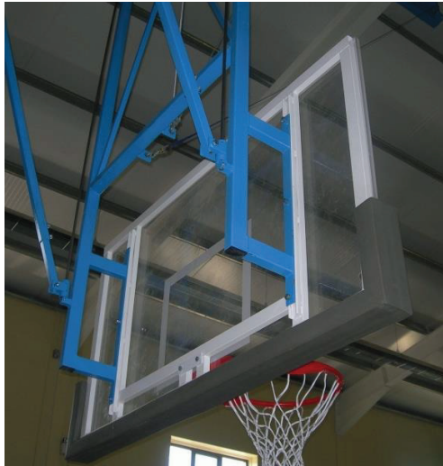
Fig. 2 Drop down goal support structure example
