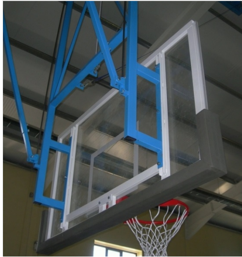
Fig. 2 Drop down goal support structure example
